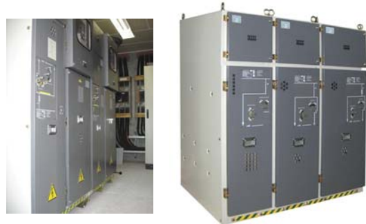
LCA-A and measurement panels. LCA-A RMU (ALBS within)
